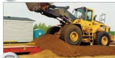
3 Backfill to bulkheads and finish ramps.
