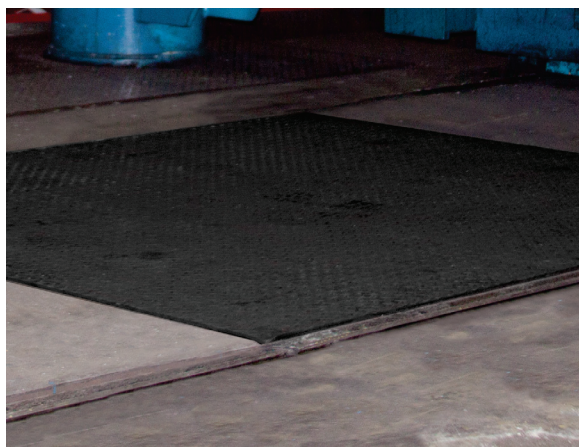
Pit mount installation
